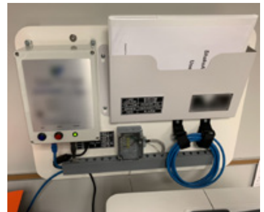
A ShakeAlert-powered box (12 in. by 16 in.) is mounted on the wall in the main office of Stanwood Elementary School in WA. The Stanwood-Camano School District has integrated ShakeAlert EEW into its public address system, so all buildings across its campus are alerted simultaneously. Image is courtesy of Varius, Inc., a ShakeAlert Licensed Operator
